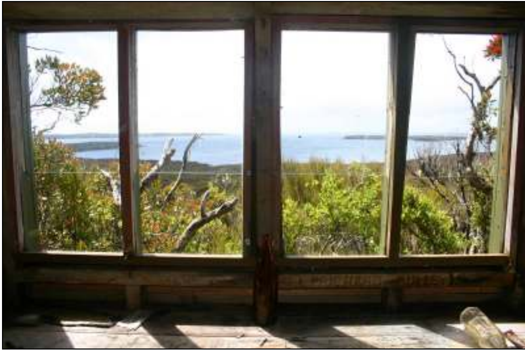
Interior of the Coast Watch Lookout Hut at Ranui
